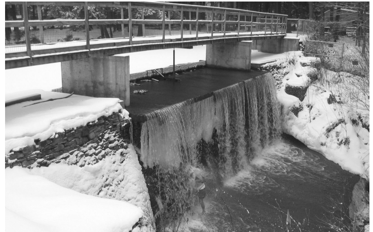
Melody Lake Dam in Cortland County is a Class C High Hazard Dam.
